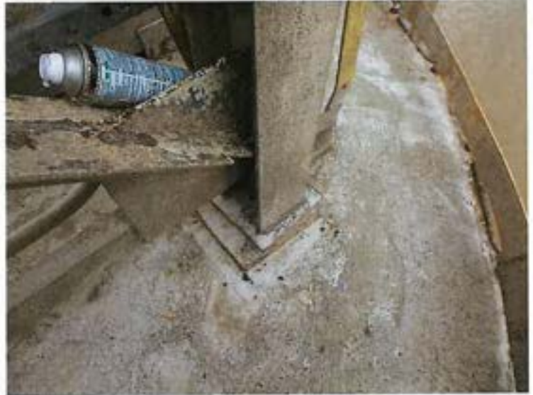
Photo 8: View of a support for the loadout conveyor.
