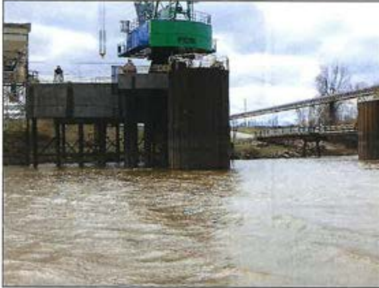
Photo 1: Elevation – Channel Side
