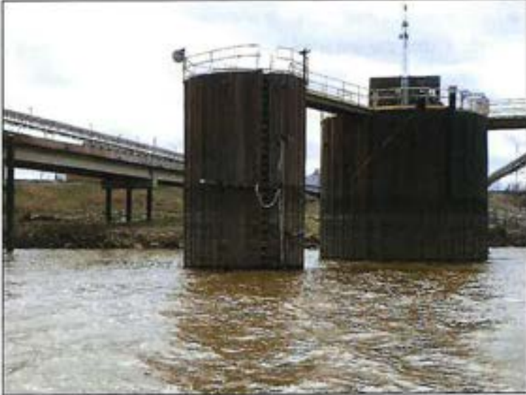
Photo 1: Elevation – Channel Side
