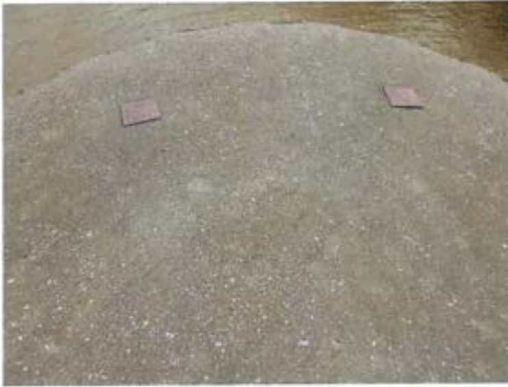
Photo 2: View of the concrete cell cap.
