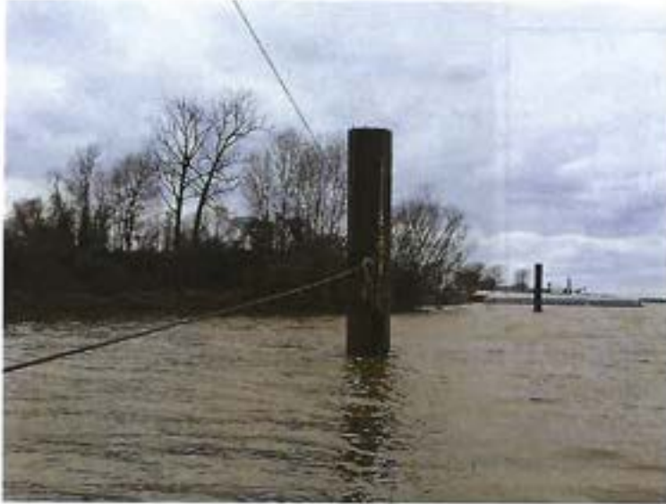
Photo 1: Elevation – Downstream Side
