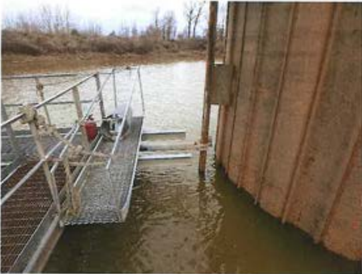
Photo 4: View of the guide pile.
