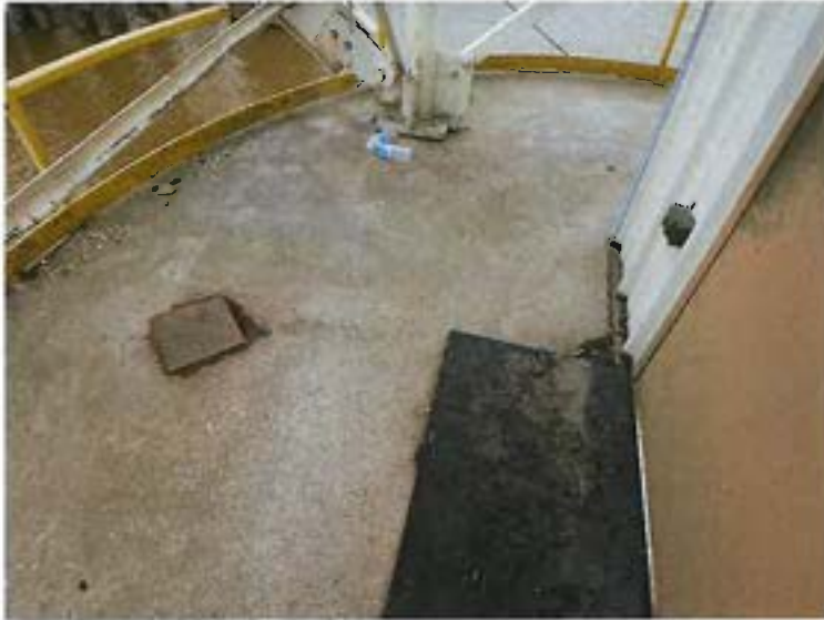
Photo 2: View of the concrete cell cap.
