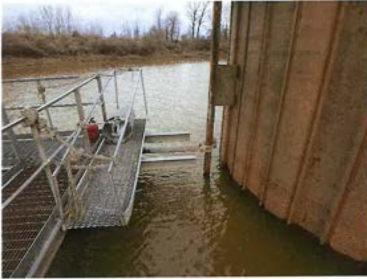
Photo 7: View of the floating dock guide pile.
