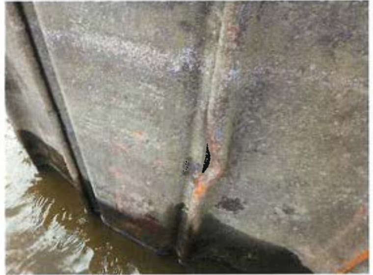
Photo 5: View of the open interlock between Sheets 3 and 4.
