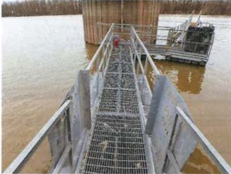
Photo 1: Elevation – View from Approach Gangway
