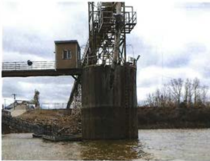
Photo 1: Elevation – Channel Side
