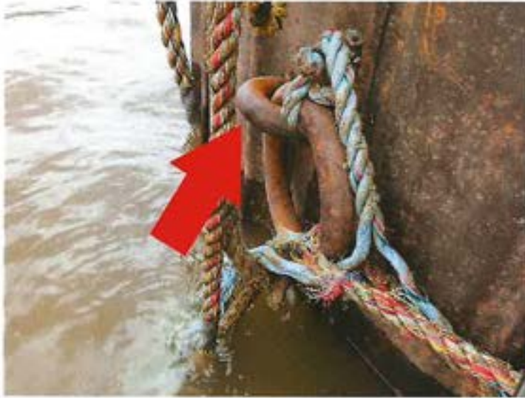
Photo 6: View of impacted U-bolt on Sheet 3.
