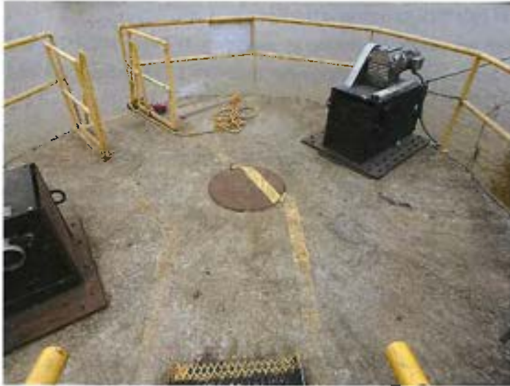
Photo 2: View of the concrete cell cap.
