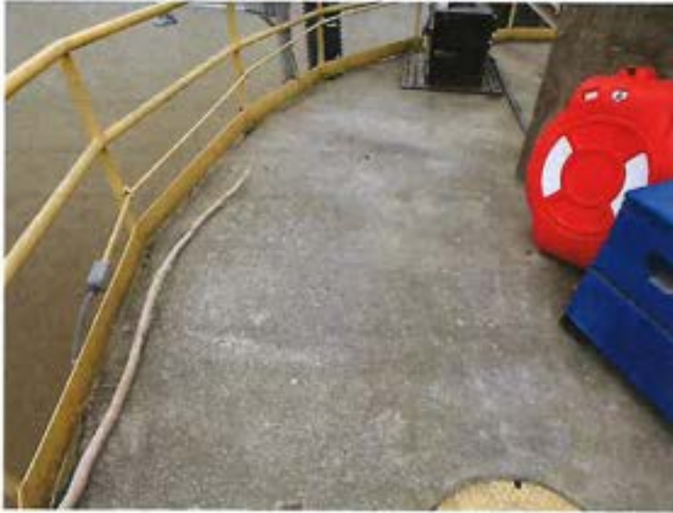
Photo 2: View of the concrete cell cap.
