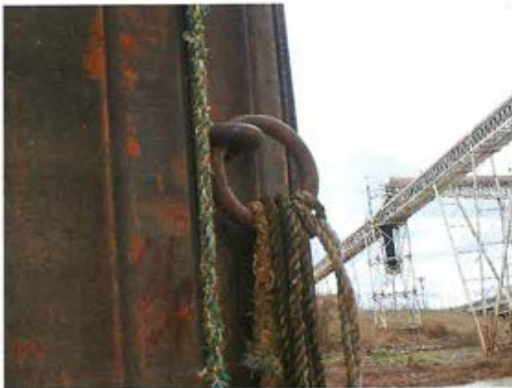
Photo 4: View of a typical mooring ring.
