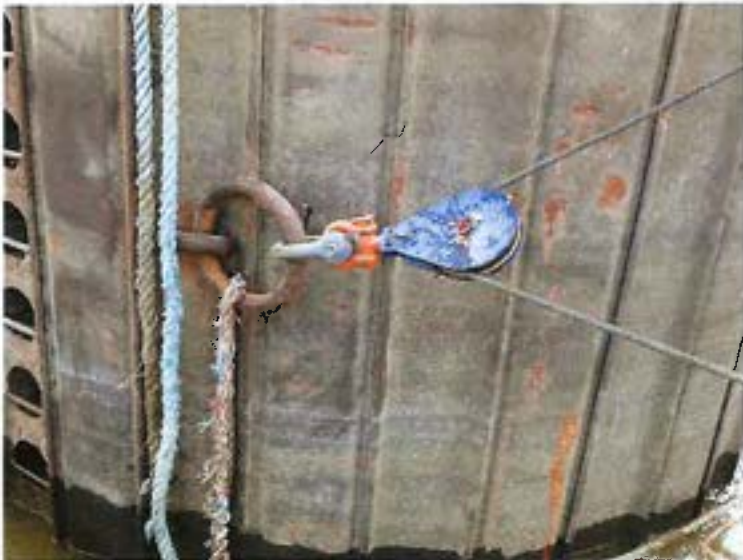
Photo 4: View of a typical mooring ring and haul line attachment.
