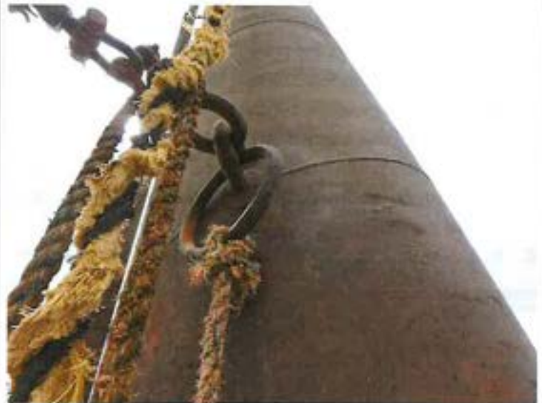
Photo 4: View of a typical mooring ring.
