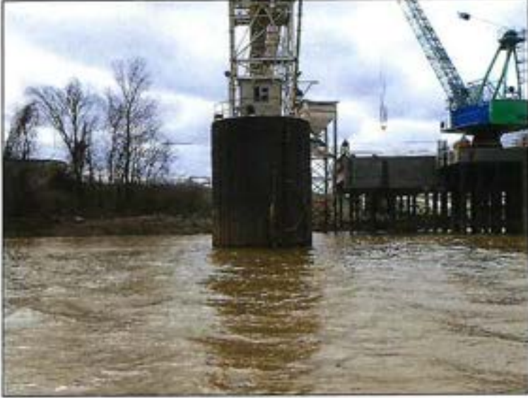
Photo 1: Elevation -- Channel Side
