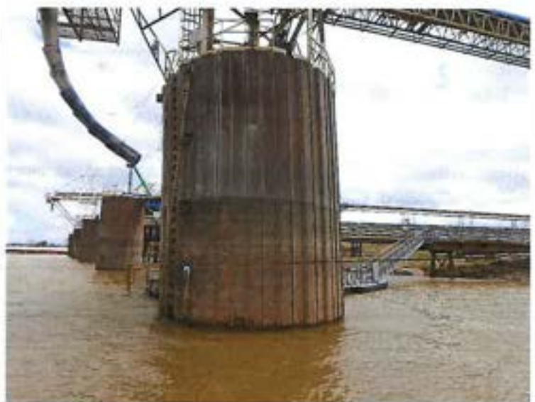
Photo 2: Elevation – Downstream Side
