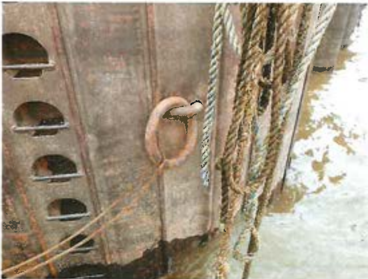
Photo 5: View of a typical mooring ring.
