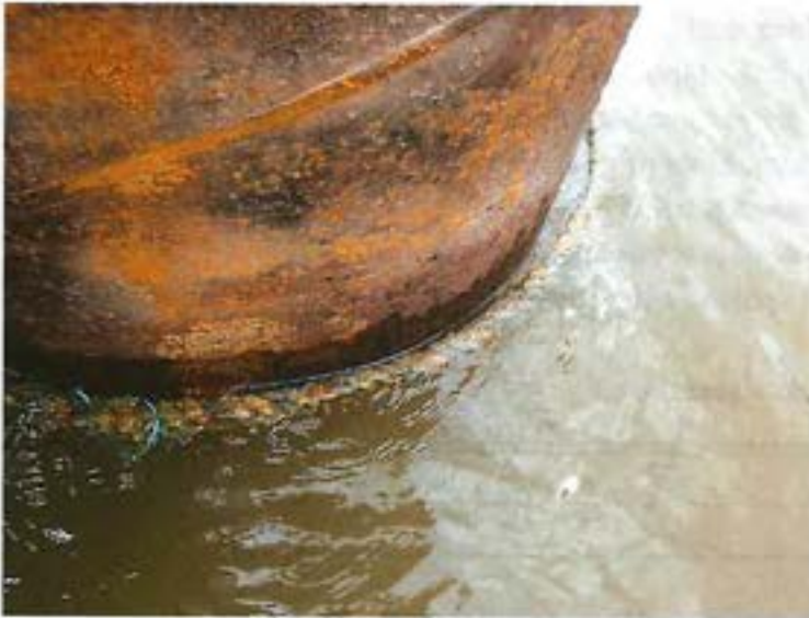
Photo 2: View of typical dolphin condition at waterline.
