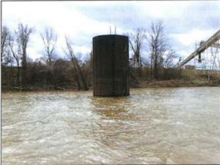
Photo 1: Elevation – Channel Side
