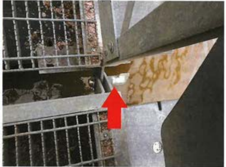
Photo 3: View of a typical keeper pin.
