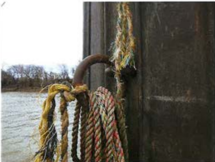
Photo 4: View of a typical mooring ring.
