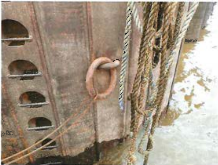
Photo 4: View of a typical mooring ring.
