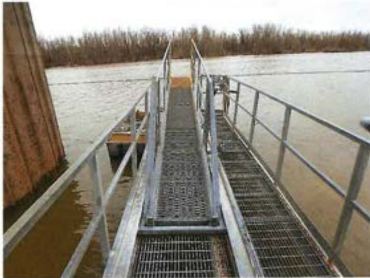
Photo 8: View of Section 3 listing to the downstream side.
