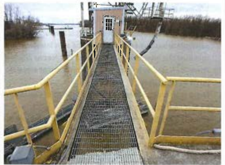
Photo 6: View of the access walkway from Cell 5.
